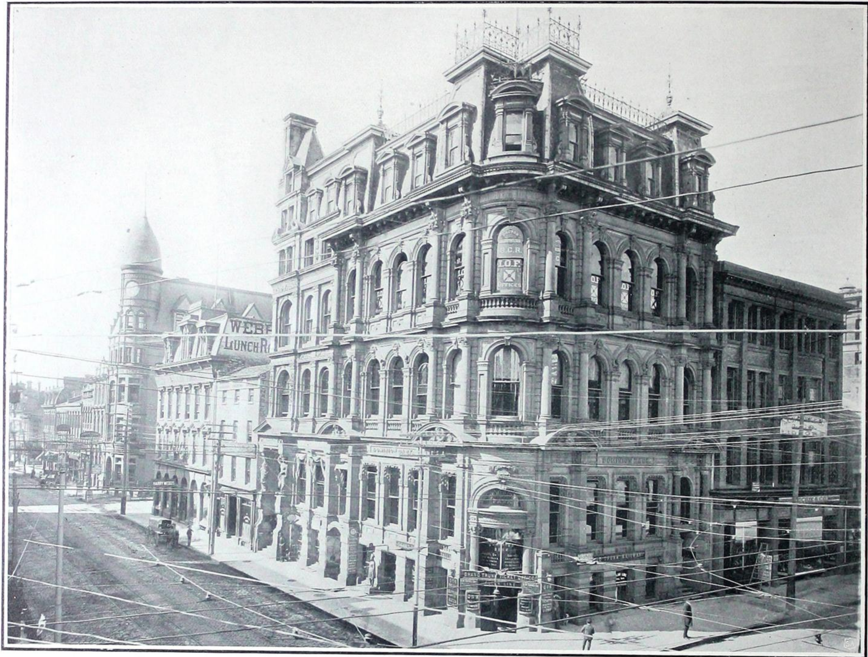
Fig. 192.—Dominion Bank, Toronto, (Head Office) In which the "Hayes" Patent Lathing was used.
